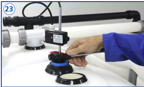
Screw on union nuts at both ends of the connecting line firmly to the tapping fittings.
