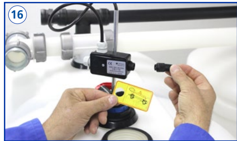
Disconnect the end plug of the overfill protection according to the tag and mount it later on the last tank.
