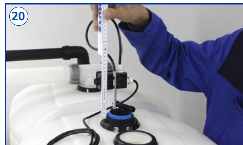
Screw the sampling extension unit tightly into the tank and check float switch setting (y dimension).
