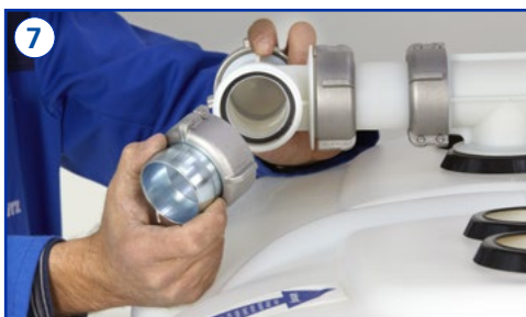
7 Connecting piece filling line (export package 2") DN 50 with the union nut to the T-piece with strainer.
