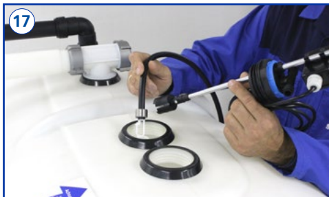
Lower the float and suction hose of the basic sampling unit into the tank.
