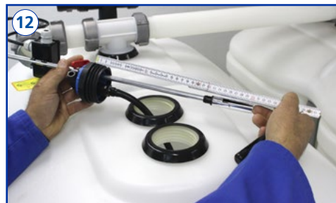
12 Set the limit value transmitter (x-dimension) according to the enclosed description.
