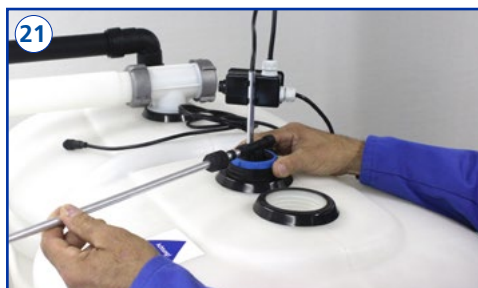
Insert connecting line with attached union nut and seal into the longer leg of the of the sampling extension unit and align at right angles to the tank.
