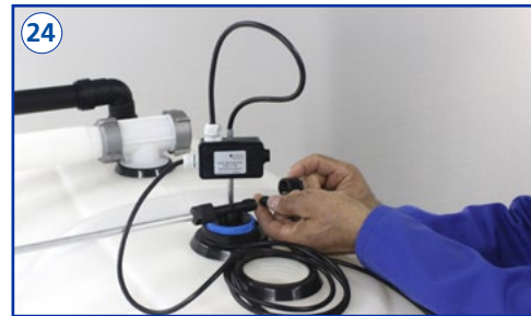
Close the last basic tapping unit with the plug and union nut.
