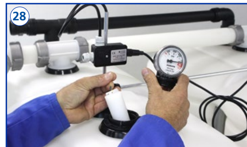
Mount content gauge with clipped-on tank scale (slowly lower the float).
