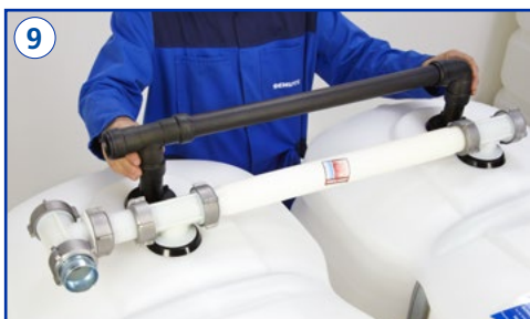
9 Pre-assemble the vent line completely and pin.
